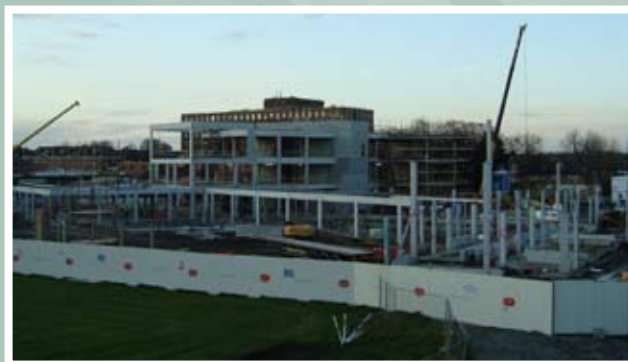
New HSE Mental Health facility
