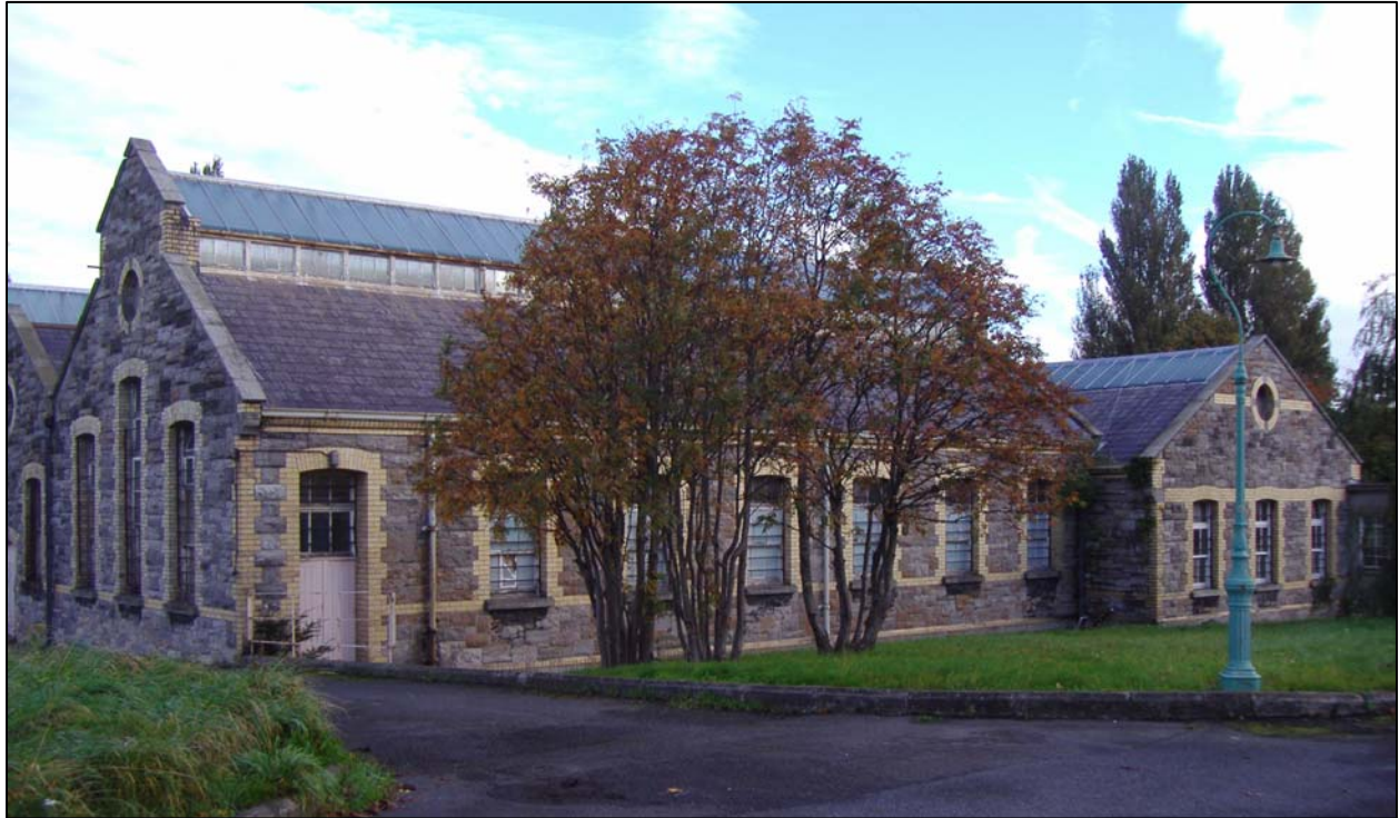
The laundry building
